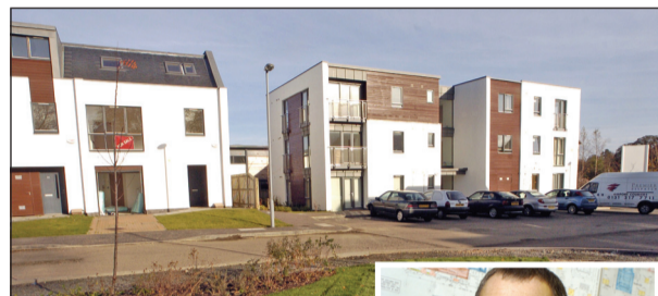
WiseBuild is nearing completion on a £1.5m project in Balerno.
